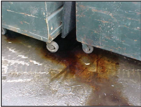
Figure 17. Leaking dumpsters can introduce pollutants into stormwater runoff.
